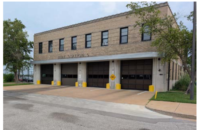
Engine House 5 New Entry Apron
