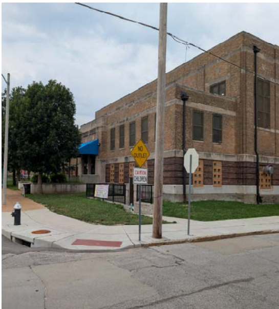
New ADA Entry for Gamble Recreation Center
