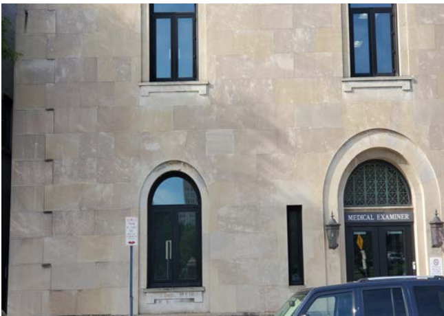
Medical Examiner Building Facade Repairs
