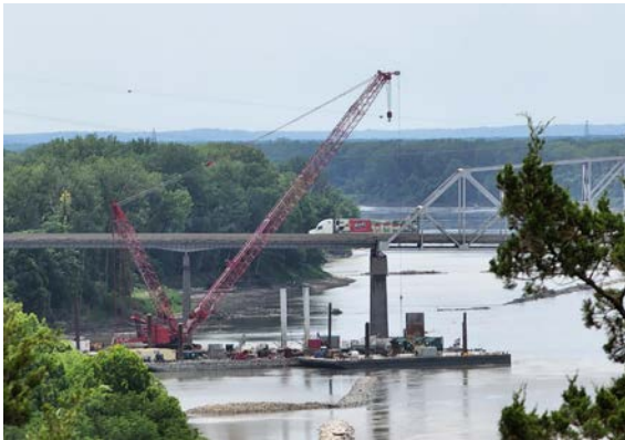
I-70 Rocheport Bridge Project
