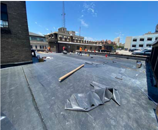
Fire Engine House Roof
